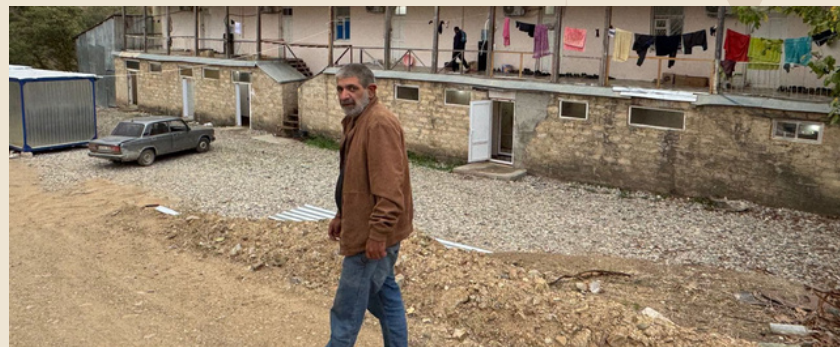
One of the refurbished buildings used to house Iranian workers coming over the border of Iran.
